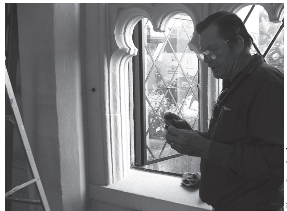
Metal Specialist Arthur Horn installs restored leaded glass window in the Ballroom, March 22, 2010.
