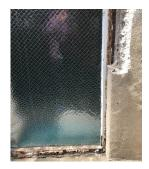
The restoration offers three glazing options: plain glass, simulated divided lights (where the diamond pattern is applied to a single pane), or true divided lights (authentic diamond-shaped panes created by welding individual glass pieces within lead came, as in the original 1929 construction). True divided lights would restore the windows to their historical authenticity and visual impact.
